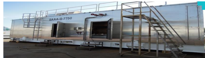
SS316L Genset Canopy
